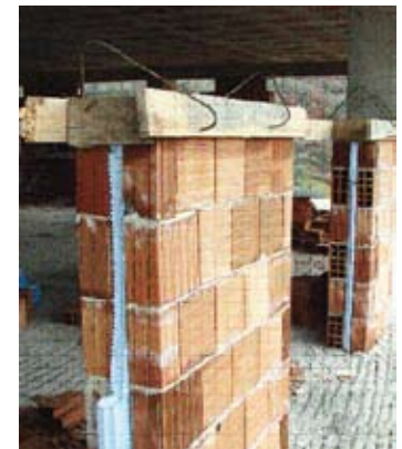
Hollësi e murit me termoizolim k = 0.874 \text{ W/m}^2\text{oK}
